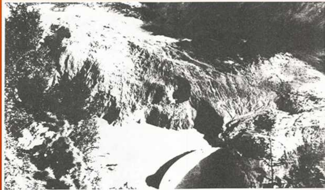
Figure 4-23.—Vaiont Dam after failure, showing massive slide upstream of dam. P-801-D-79375.
