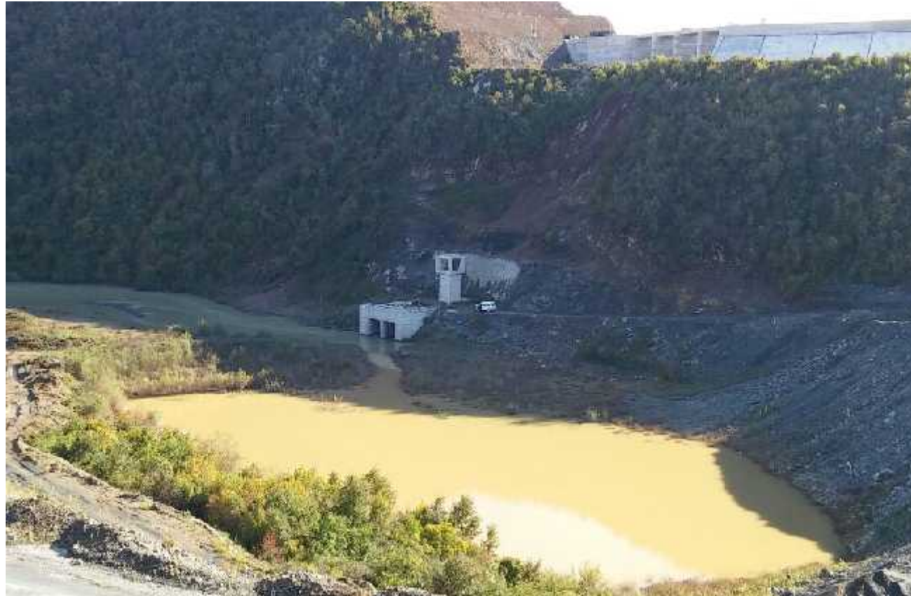
Fan River Hydro Power Project, Aydiner Construction Co., Lezhe, Albania
