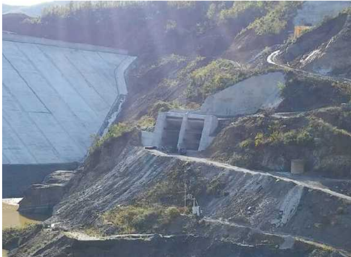
Fan River Hydro Power Project, Aydiner Construction Co., Lezhe, Albania
