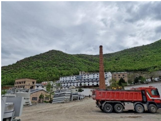
Figure 10 - Chrome mining factory in Bulqize, in operation since 1972.
