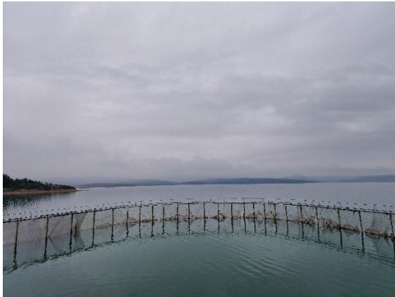
Thana Reservoir: the largest artificial reservoir in Albania.
