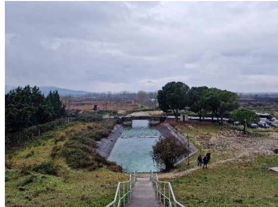
Main irrigation channel downstream of the dam.
